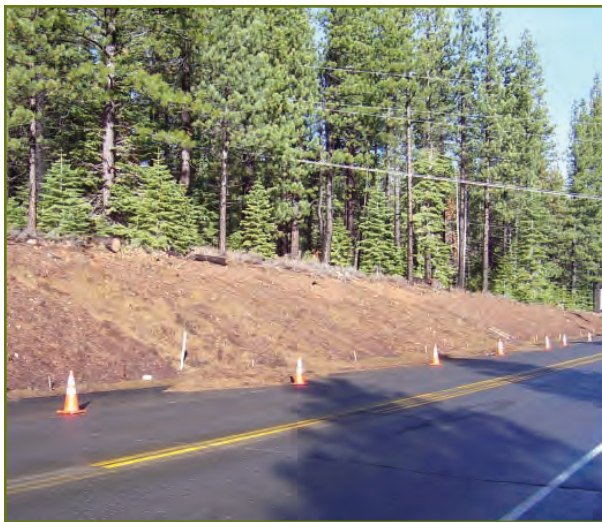
Slope failures following large storm event – December 2005.
