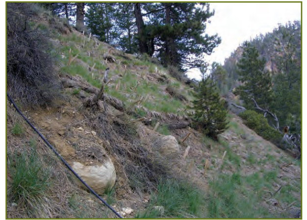
6- Project site one year after treatment.
