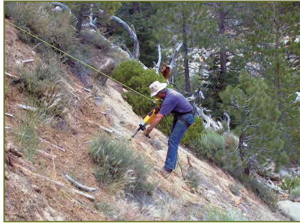
2- Drilling holes in slope with hammer drill.
