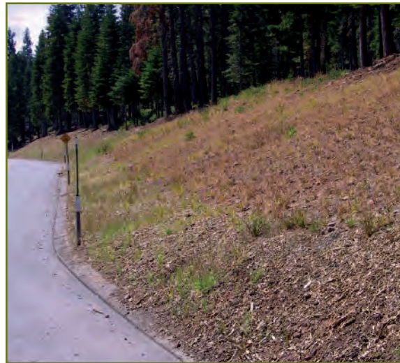
Contiguous slopes at Northstar Unit 7 in 2006 — hydroseeding treatment (left); full soil treatment (right).
