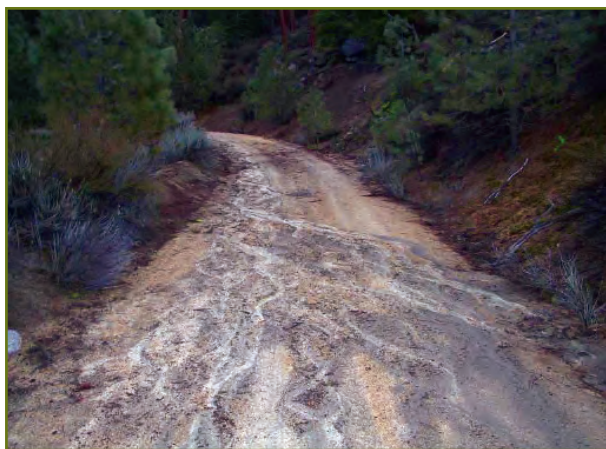
Erosion on dirt road.
