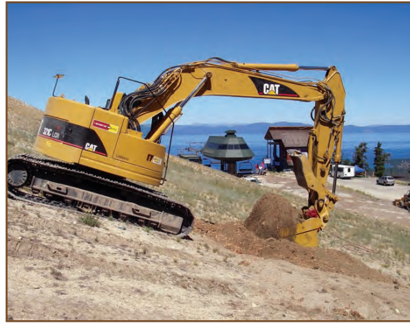
Tilling has proven to be a highly effective method for loosening dense soil and incorporating organic matter.
