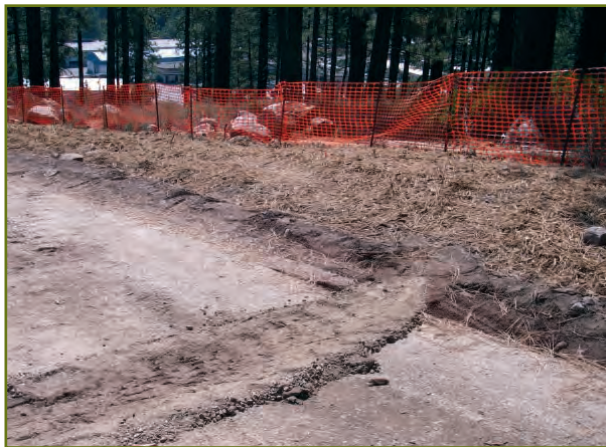
Re-disturbance of unprotected roadside treatment areas is a common problem.
