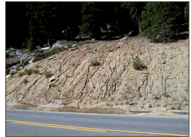
This road cut exhibits evidence of high runoff and erosion resulting from lack of infiltration capacity and vegetation.
