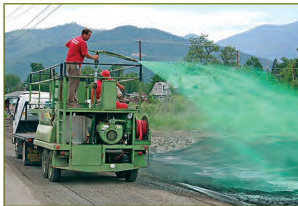
Seed application methods – hand seeding (left), hydroseeding (center), drill seeding (right).
