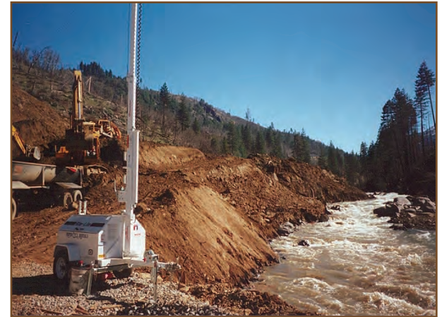
This photo of the American River shows a mass failure that temporarily blocked the river. This slide was believed to be the result of lack of vegetation from a previous fire, defoliation efforts, and water associated with a 100-year precipitation event (1997).
