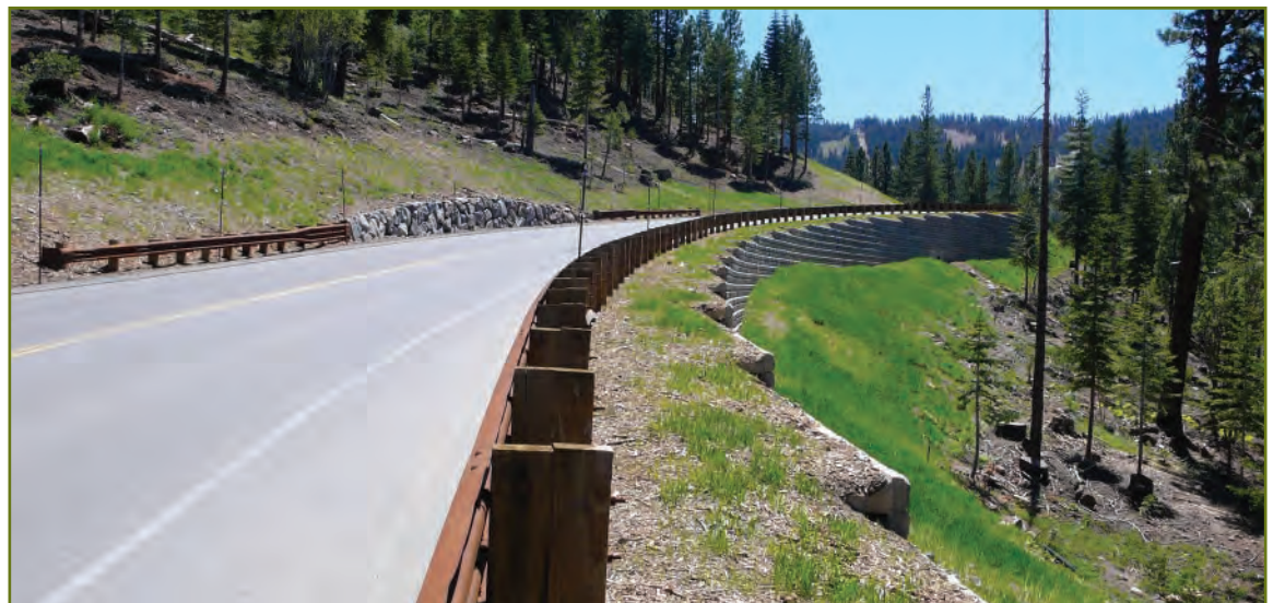
Highlands View Road at Northstar-at-Tahoe, one year following treatment. Topsoil was salvaged and re-applied along 4 miles of cut-and-fill slopes.
