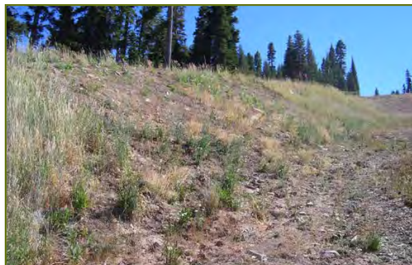
Northstar Superpipe – failure caused by over-irrigation (top); repaired slopes with proper irrigation (center); stabilized slopes two years after treatment (bottom).
