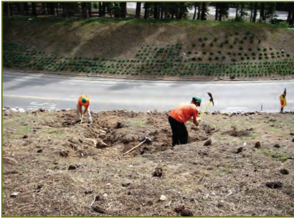
Loosening soil by hand using pick mattocks.
