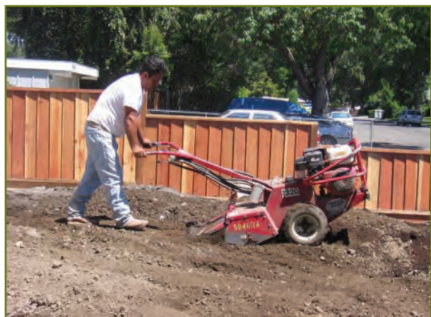
Loosening soil with hand-operated rototiller.
