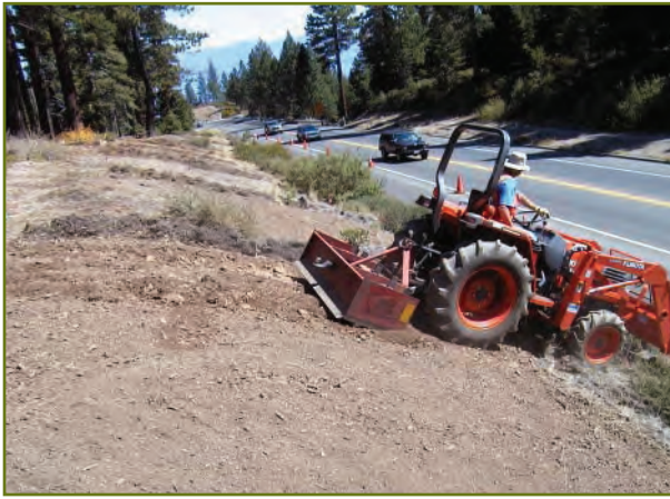
Tractor-mounted subsoiler being used to mix amendments into soil.
