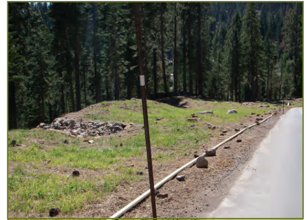
Infiltration areas off Highlands View Drive at Northstar-at-Tahoe. Full soil-vegetation treatment was implemented to maximize infiltration over the entire roadside. In addition, berms were constructed every 50 feet to direct high flows to stable, rock-armored outfall areas.
