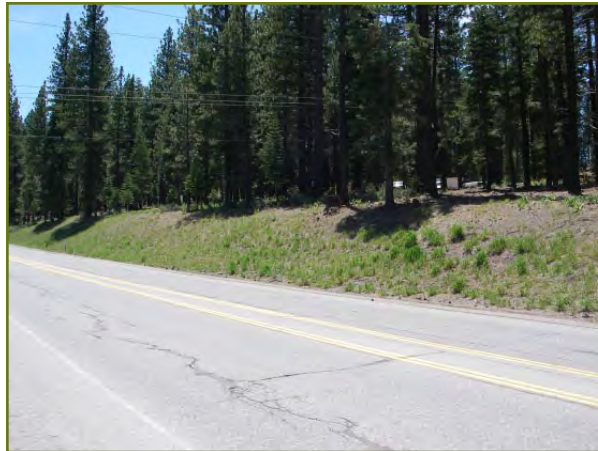
Highway 267 slope, three years after treatment.
