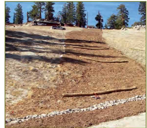
Test plots were integrated into this post-construction restoration treatment following installation of a waterline at Heavenly. The treatment area was simply divided in half and two different soil amendments were used.
