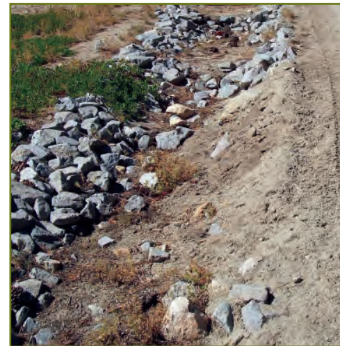
Deposited sediment in unmaintained rock-lined ditch.
