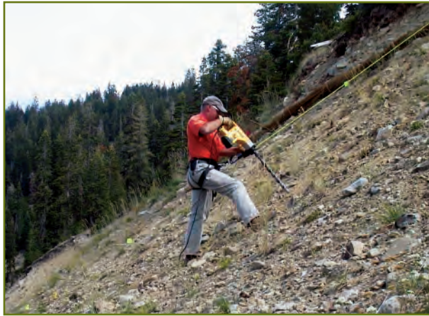
Drilling holes using hammer drill to increase infiltration on extremely dense cut slope in Squaw Valley.
