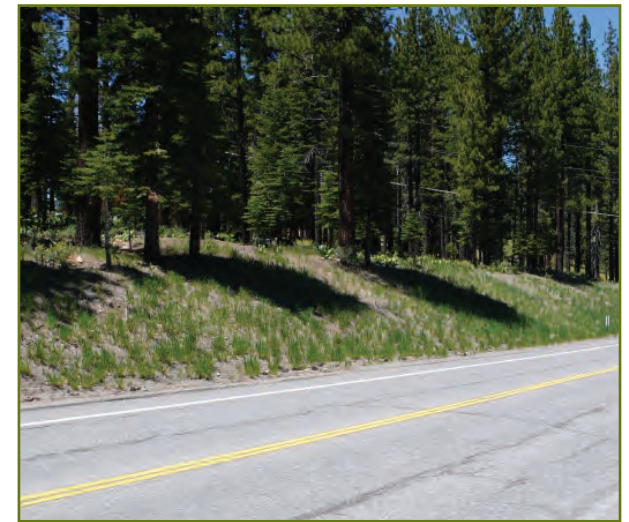
Repaired slope exhibiting long-term stability – Summer 2008.
