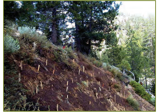
3- Wooden stakes were hammered into slope to increase infiltration and provide anchors to hold compost in place.
